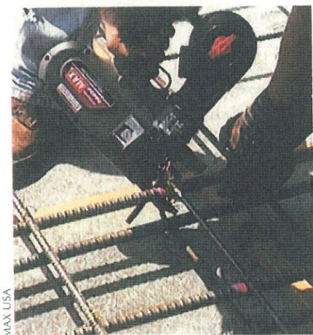
Figure 4. A mechanical rebar tie gun can make a secure connection in less than a second.
