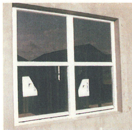
Figure 6. Windows are installed from the outside of the wall and are pressed into a continuous bead of silicone sealant against a 7/8-inch offset lip cast in the opening. The installation tolerance is tight, typically only about 1/4 inch over the unit dimension, to minimize air infiltration around the window.
