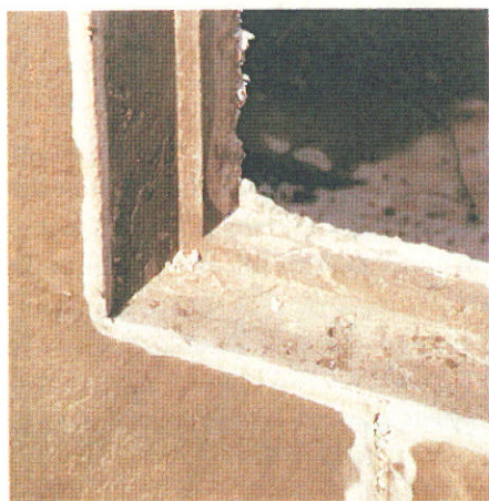
Figure 6. Windows are installed from the outside of the wall and are pressed into a continuous bead of silicone sealant against a 7/8-inch offset lip cast in the opening. The installation tolerance is tight, typically only about 1/4 inch over the unit dimension, to minimize air infiltration around the window.
