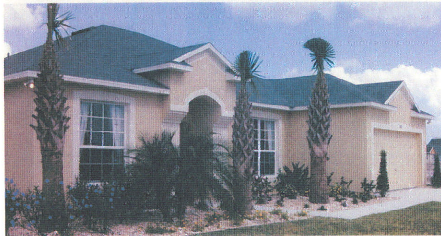
Figure 10. One-coat stucco and standardized decorative detailing provide a simple, attractive, and durable exterior finish.
